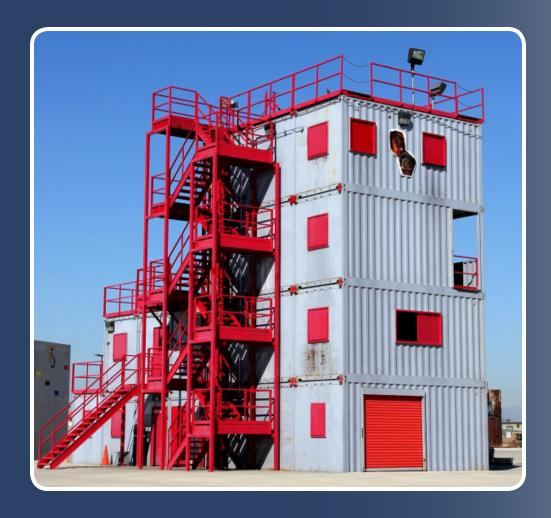
Our Four Story Expandable Training Tower provides 4160 square feet of interior training space. The unit is equipped with a flat and pitched roof, exterior decks on two levels and a balcony across the front of the entire structure. The facility includes an interior staircase to each level and provides two burn rooms for live fire training. The roof includes safety rails and two cutting locations.
